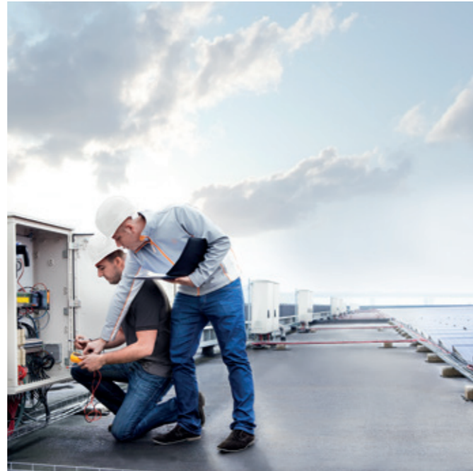
In case of complex photovoltaic systems, faults and loss of performance often go unnoticed for a long time. Transclenic 16i+ 1k5 facilitates monitoring and thus raises performance.
